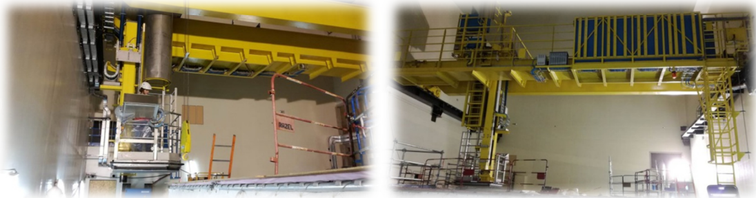
Fig. 6: One-site pool crane commissioning tests
